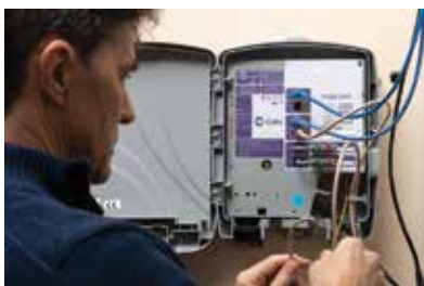
Hooking up service at the home.
